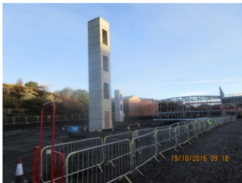
Photographs 7 and 8 Lift Shaft No 2 in October 2016 and now encased March 2017
