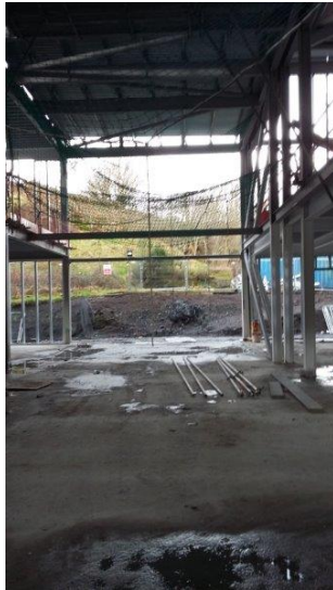
Photograph 9 The double height main entrance
