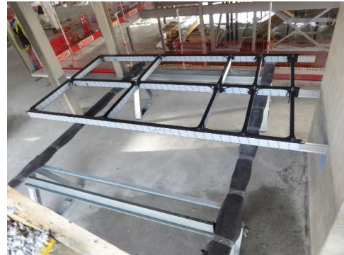
Photograph 10 Glazed screen elements assembled on site
